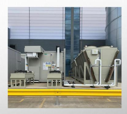
There was a restriction to the plant area footprint, so it was important to ensure the external equipment design was suitable. For this reason, a V-block gas cooler was selected.
