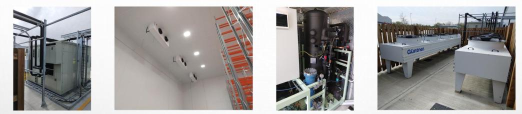
Each system was connected to a  $CO_2$  Guntner Gas Cooler. Both were oversized to cope with extreme conditions and has increased corrosion protection to extend the life of the equipment.
