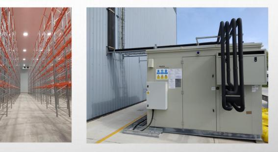
Each of the ECO2 MAXI 4×0 HT compressor packs had 3no Bitzer 4GTE-20K and 1no Bitzer 4GTE-30k compressors. Both packs were supplied within a housed walk-in.
