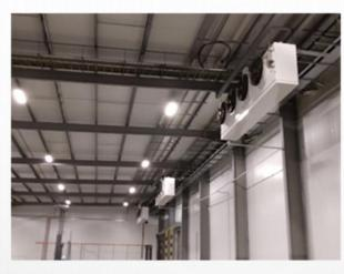
Based on the client's requirements, the Kelvion evaporators have a 5K TD between room and evaporating temperature.
